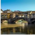
The Pont Vecchio is a medieval stone bridge in Florence, built over the Arno River. Its location, closed-spandrel segmental arch shape
